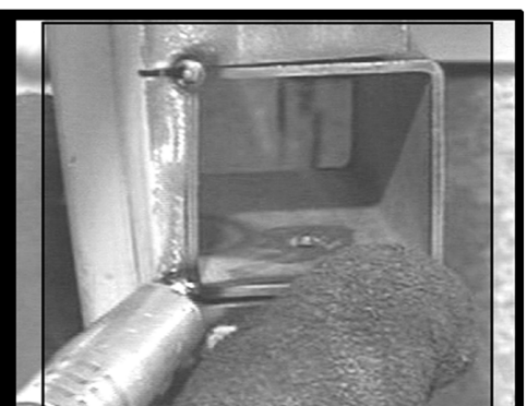
Tack tubes on two outer corners only then check alignment.
